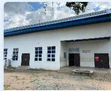
MICTU Building Management Information Communication and Technology Unit.
