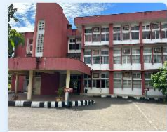
Administrative Block A Main administrative building -
